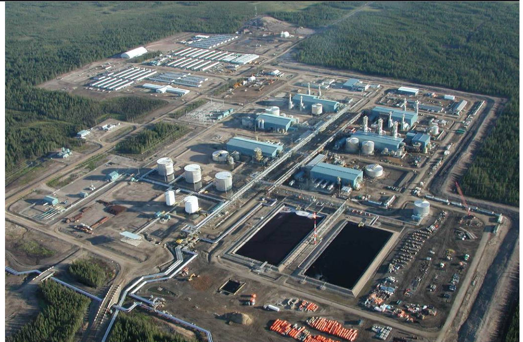
Suncor Energy's Firebag I and II SAGD facilities
