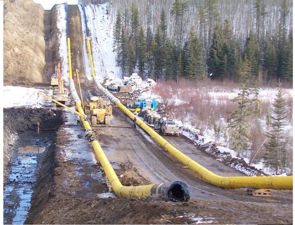
Pipeline installation, river crossing, N.E. Alberta
