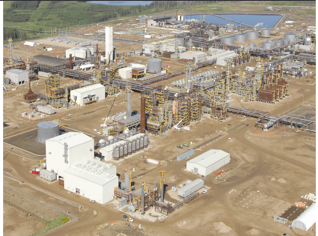
Nexen-Opti's Long Lake - Flint built the project's Gasifier Unit
